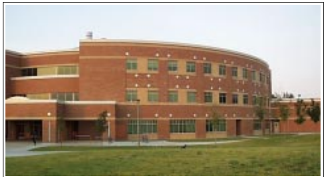
Location of the Burns Telecommunication Center on the campus of MSU-Bozeman
